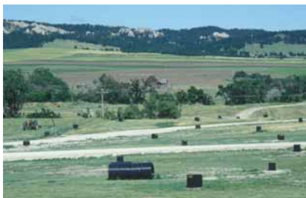
A typical ISR uranium mine
