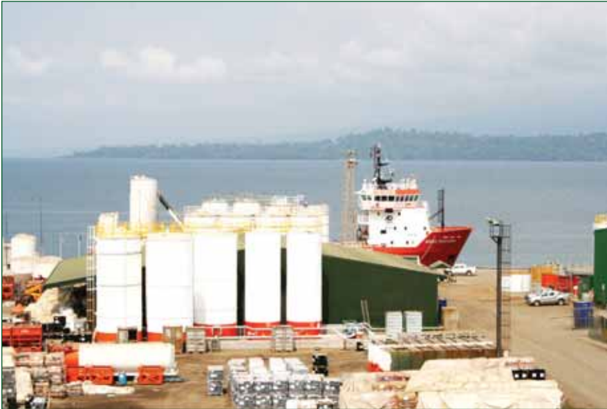
Freeport project, Luba mud-drilling facility
